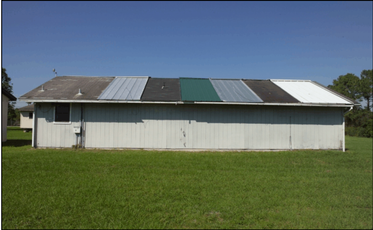
Figure 4. Flexible Roof Facility in summer of 2004 configuration
