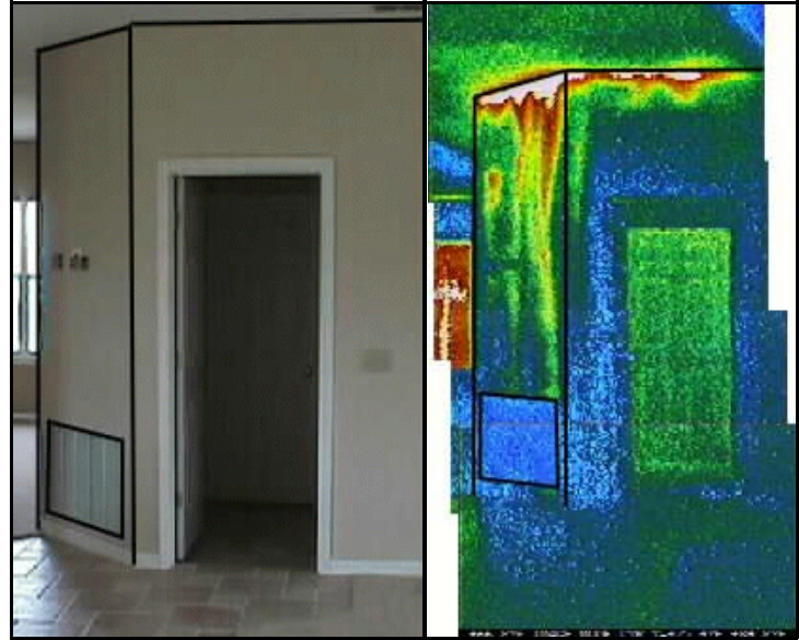
Figure 2. Thermograph of air being drawn from the attic to the air handler in a Florida house.
