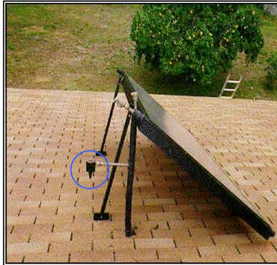
Figure 1.3-8. Freeze valve jutting from collector return line.
