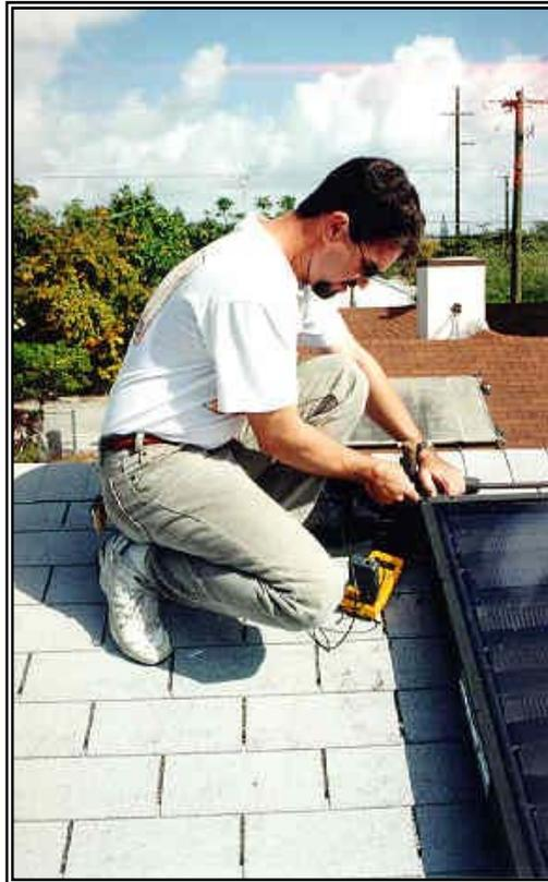
Figure 1.8-2. Shawn Angell of the Metro-Dade Community Action Agency checking a collector sensor.
