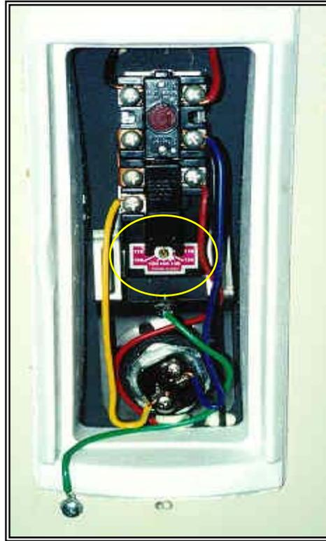
Figure 1.3-15. Water heater thermostat.
