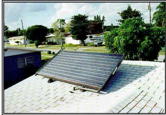
Figure 1.3-5. Flat-plate collector mounted at an angle.
