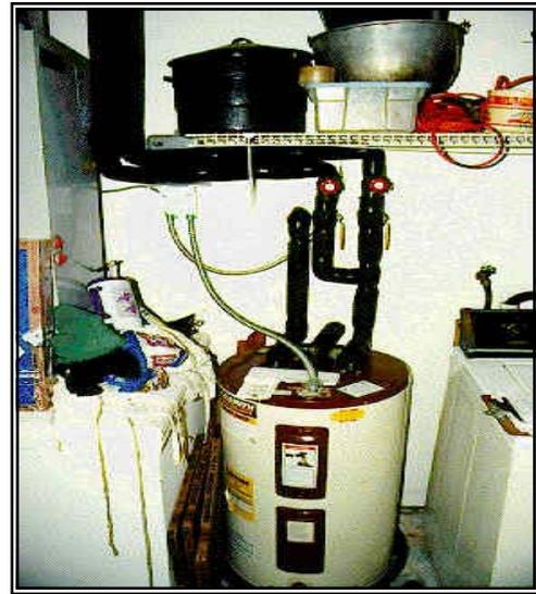
Figure 1.3-2. Water heater and plumbing from ICS system.
