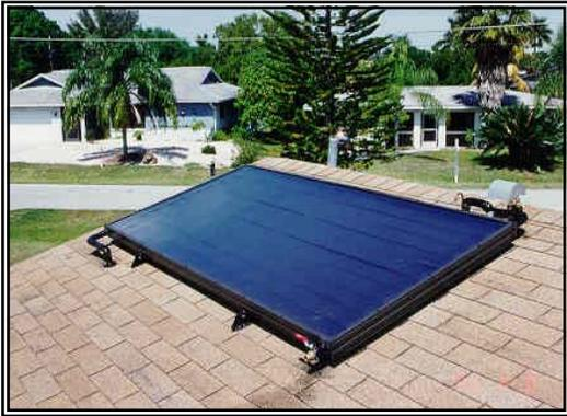
Figure 1.3-4. Flat-plate collector mounted flush to roof.
