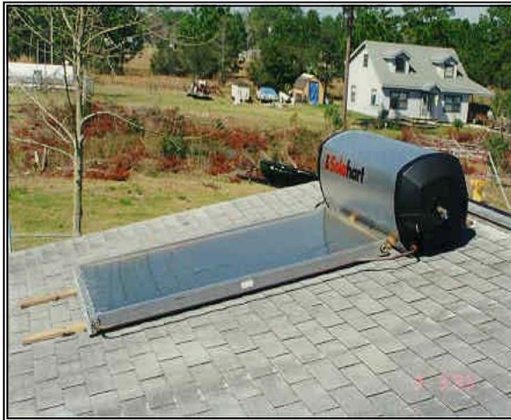
Figure 1.3-3. Thermosiphon system in Central Florida.
